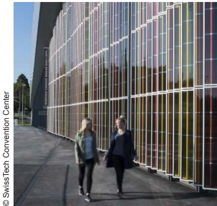
Abb. 4.3.4-04: DSC-Sonnenschutzlamellen, Swisstech Convention Center, Lausanne
